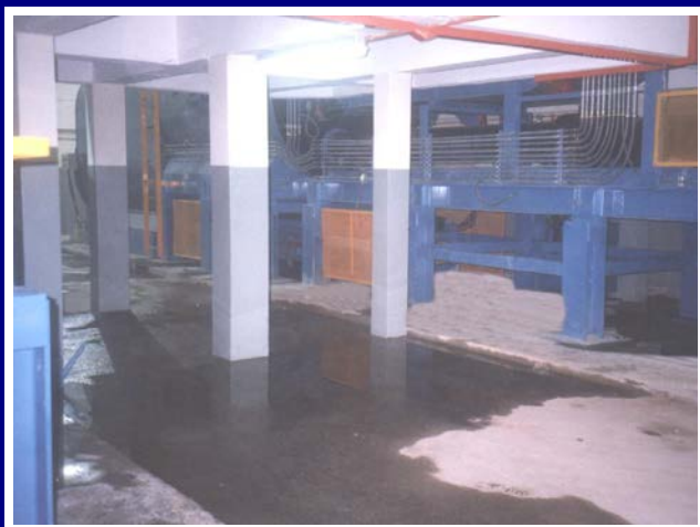
← View below mezzanine waste tipping floor
